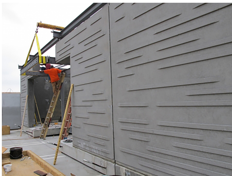
Kuva 5. The University of North Carolina at Charlotte on tutkinut geopolymeeriä rakennusmateriaalina UrbanEden-projektissa. Kuva: UNC Charlotte (2016). The University of North Carolina at Charlotte has researched geopolymer as construction material in UrbanEden-project. Photo: UNC Charlotte (2016)
